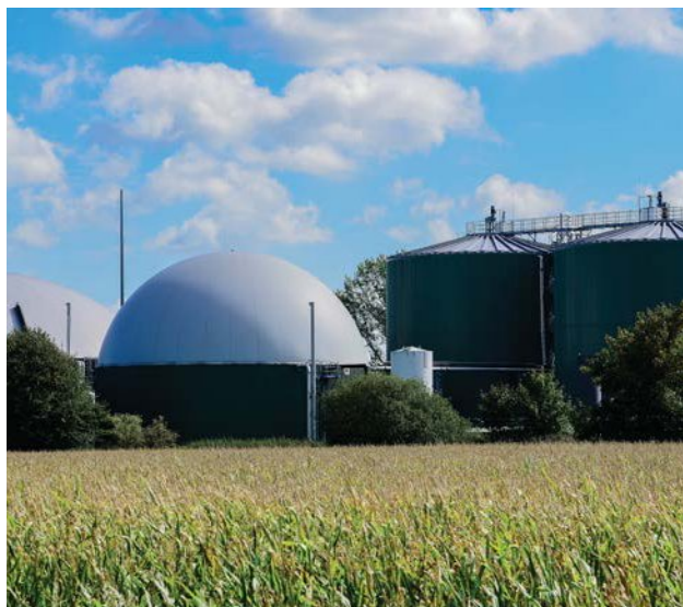
FIGURE 4 A biogas generator
