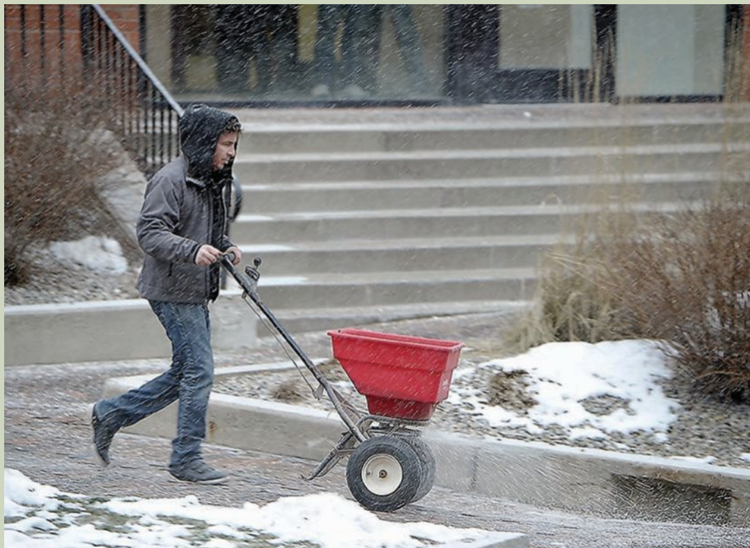
Figure 4B–1 Calcium chloride is spread on an ice-covered road to lower the freezing point of water.
