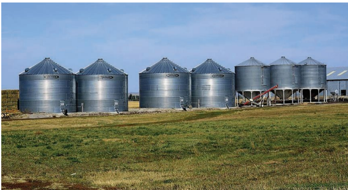
Figure 12D–2 Grain storage bins made of galvanized steel are a common sight in Australia.
