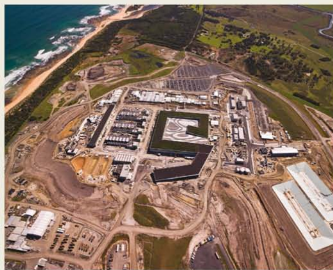
FIGURE 17.1.8 Desalination plant at Wonthaggi, Victoria.
