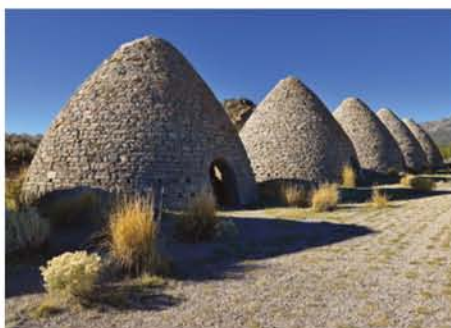
FIGURE 8.1.14 These ovens in Nevada, USA, were built between 1876 to 1879 to make charcoal.
