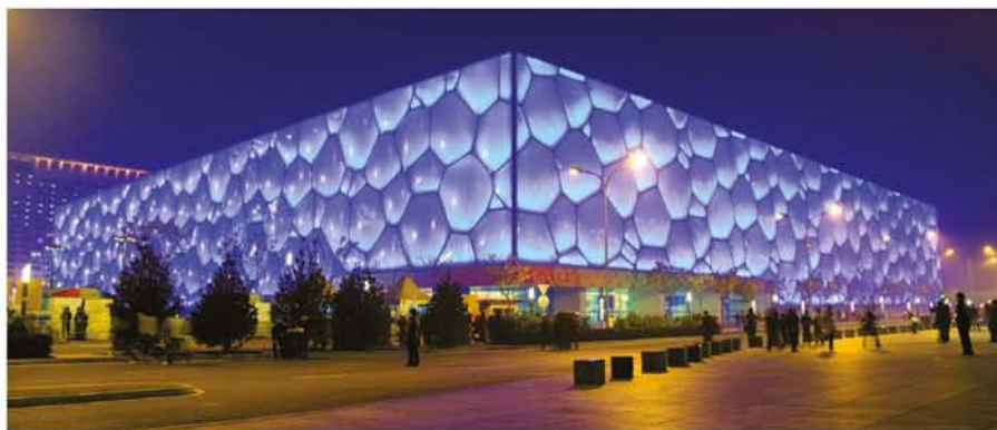
FIGURE 10.2.5 The outer shell of the Water Cube Stadium in Beijing, China, is made of ETFE, a new copolymer building material.
