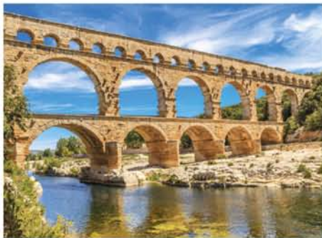
FIGURE 17.1.1 The Pont du Gard is an aqueduct in France built by the Romans in the first century. It stands 49 metres high and was 50 km long. The aqueduct carried water from a spring to the town of Nimes.
