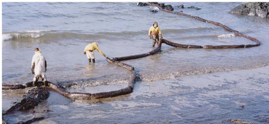
FIGURE 19.1.8 Booms are used to protect the coast from an oil spill.
