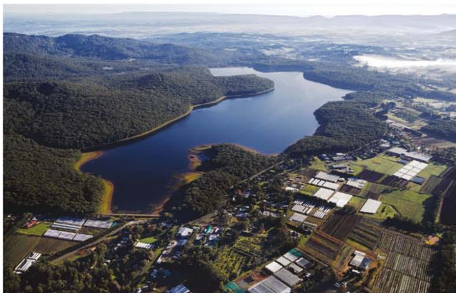
FIGURE 17.1.5 The Silvan Reservoir stores water from the Upper Yarra, Thomson and O'Shannassy reservoirs for Melbourne's water supply. Note the surrounding protected land.
