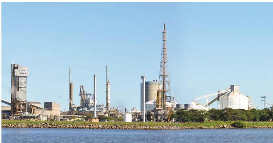
FIGURE 8.7.2 Orica produces ammonia at its Kooragang Island plant in New South Wales. It also produces nitric acid and ammonium nitrate.
