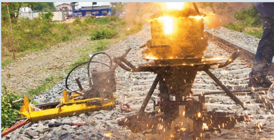
FIGURE 5.3.2 Thermite welding of railway tracks.
