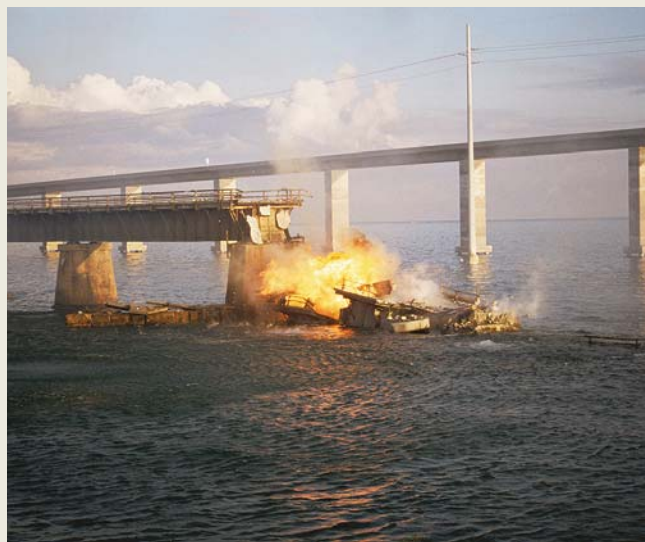
FIGURE 2.2.3 An old bridge is demolished with the help of explosives.
