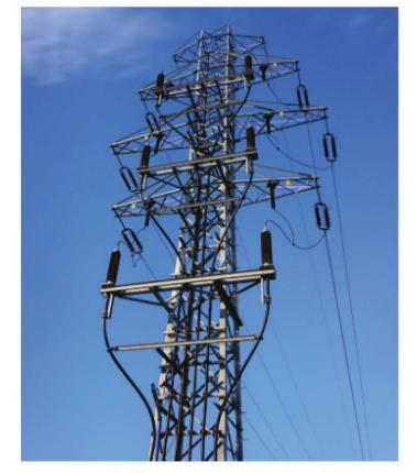
FIGURE 4.1.3 This power transmission tower relies on the strength of iron in steel for its structural integrity. The electricity cables are made from aluminium, utilising its ductility and electrical conductivity.
