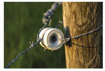
FIGURE 5.1.10 A ceramic insulator on the post of an electric fence
