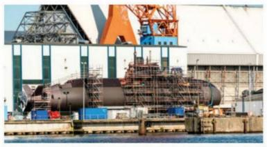
**FIGURE 5.3.4** Type 212 class submarines are being constructed for the German and Italian navies. They use proton-exchange membrane fuel cells that operate on compressed hydrogen. The submarines can remain submerged for up to 3 weeks and are very quiet and virtually undetectable.
