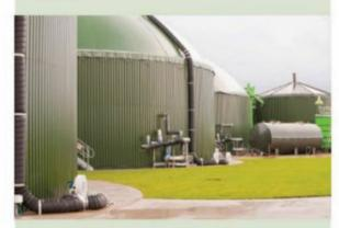
Large digestor tanks similar to those used at Berrybank Farm for biogas production
