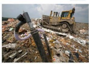
FIGURE 2.2.12 Pipes buried in this rubbish tip collect biogas.
