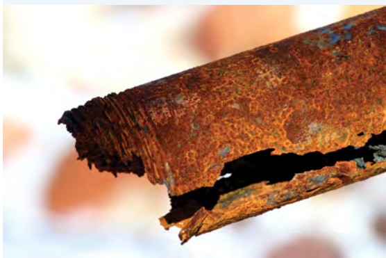
FIGURE 14.13 Corrosion of an iron pipe
