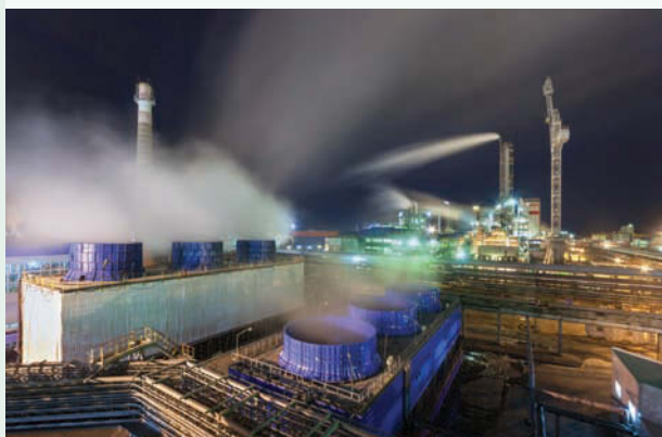
FIGURE 6.14 Production plant for ammonia and nitrogen fertilizer. Note the large cooling towers.
