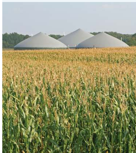
FIGURE 7.35 Maize used as a renewable feedstock, with a biogas plant in the background
