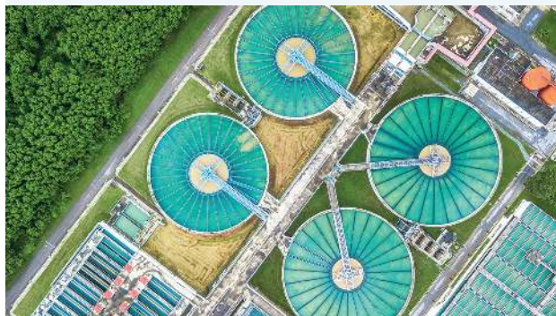
FIGURE 13.8 Water treatment plants contain large tanks that allow precipitates and other solid material to settle.
