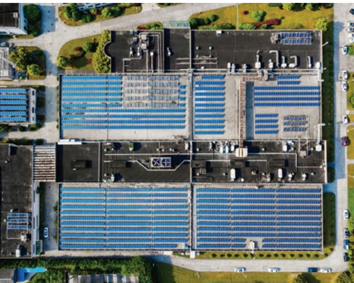
Figure 6.26: Installing solar panels on factory rooftops is one strategy implemented by food processing and manufacturing industries to reduce their environmental impact.
