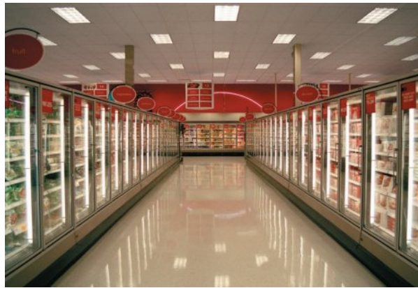
Self-closing refrigerator cabinets are more energy efficient than open refrigerated displays.
