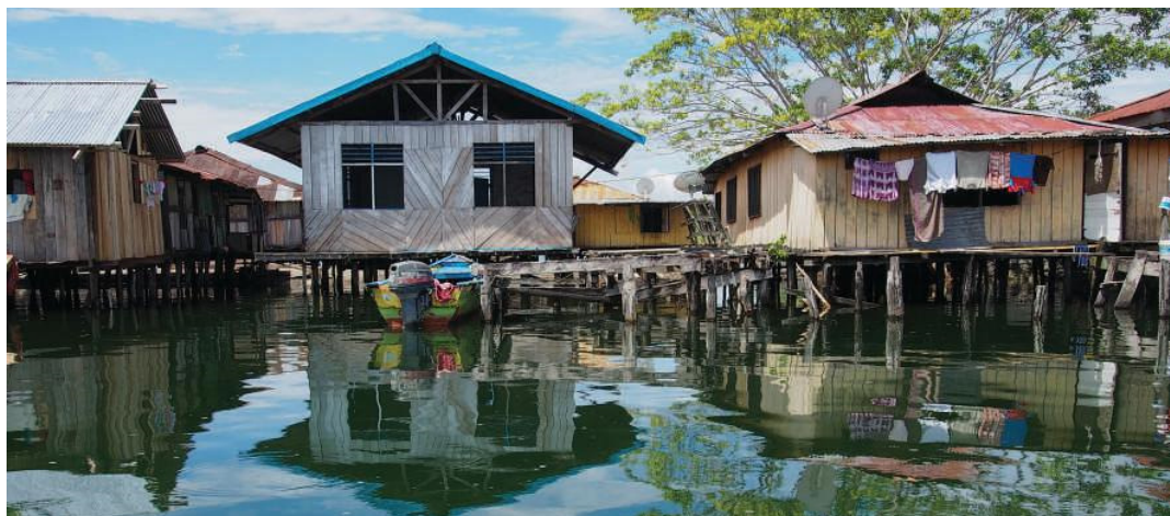
► Figure 4.36 High-density housing on stilts in Sumatra, Indonesia
