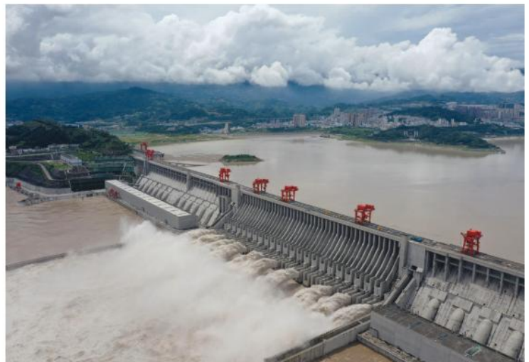
Figure 4.43 Authorities were forced to release floodwater from the Three Gorges Dam at a rate of up to 48,000 cubic metres per second in order to prevent a dam breach and a further catastrophe
