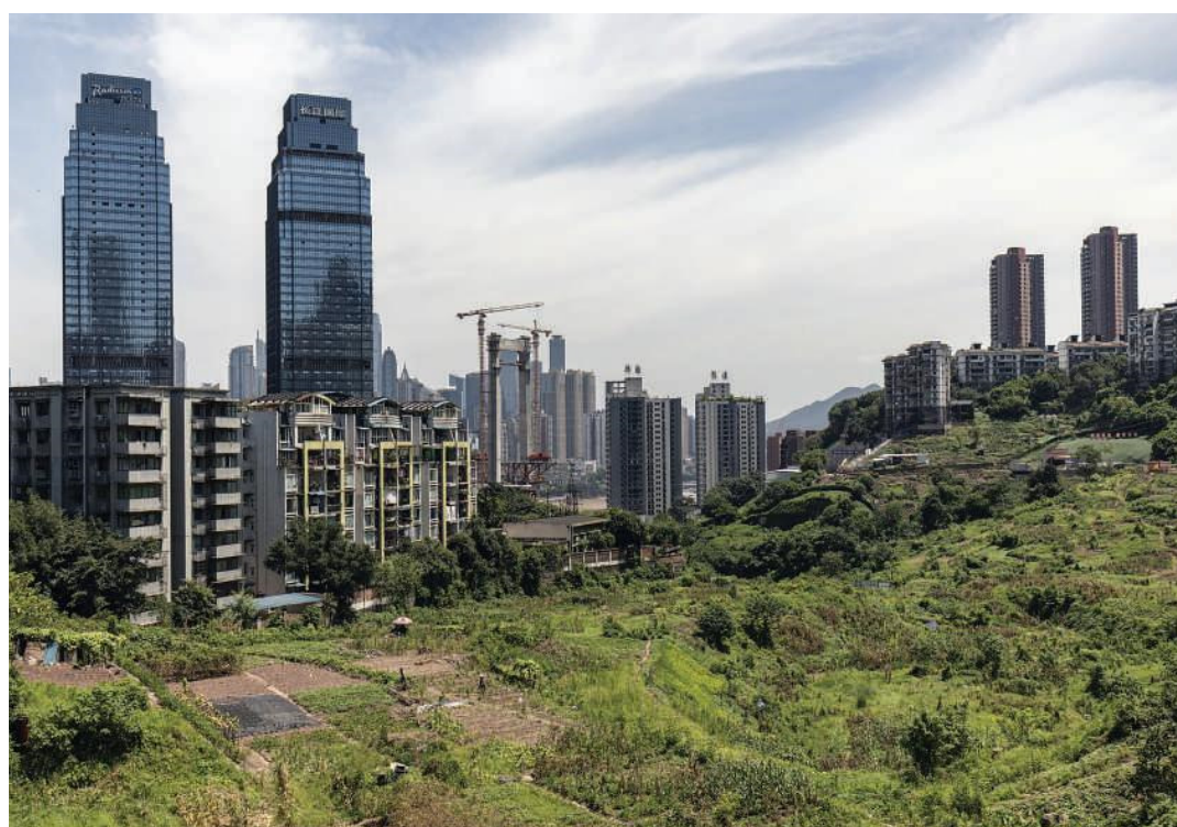
▲ Figure 4.40 Sponge cities, such as the district of Yuelai in north-eastern Chongqing, are designed to soak up heavy rainfall and release it slowly into local waterways
