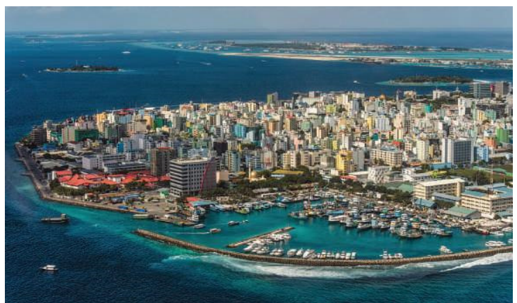
▲ Figure 2.25 Male is Maldives' capital city and is protected from ocean-based hazard events by extensive three-metre-high walls
