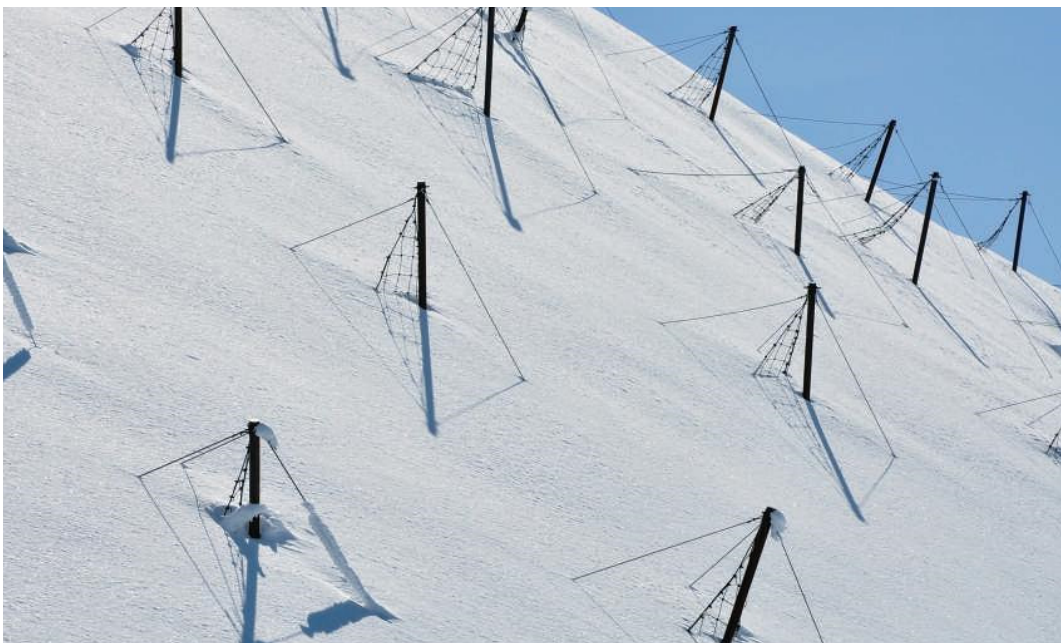
◀ Figure 3.41 Avalanche barriers protecting ski slopes in Kitzsteinhorn Alps, Austria
