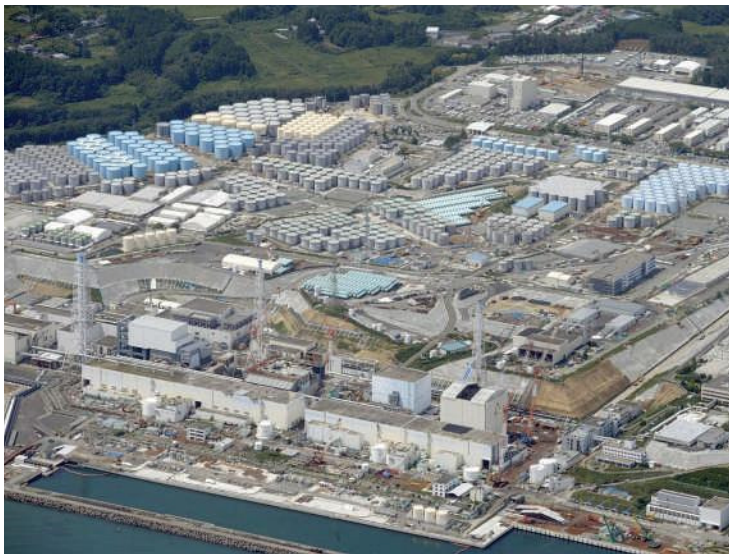
▼ Figure 6.32 Storage of radioactive waste water in large tanks on site at the crippled power plant
