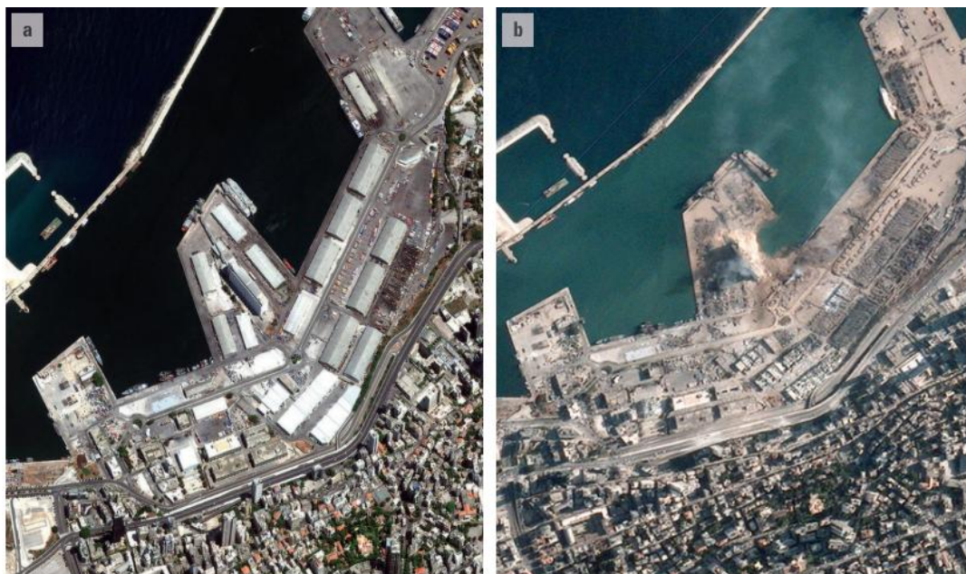
▲ Figure 1.14 Satellite images of the port of Beirut, Lebanon before and after the August 2020 explosion
