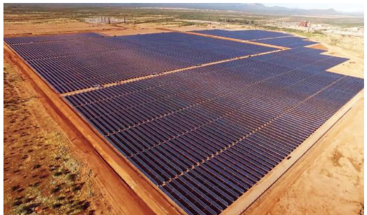
▲ Figure 2.24 Part of Morocco's drive to achieve 50 per cent renewable energy by 2040 is developing solar energy plants
