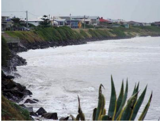
▼ Figure 4.30 The erosion at East Beach is removing the sand and risking the destruction of adjacent houses
