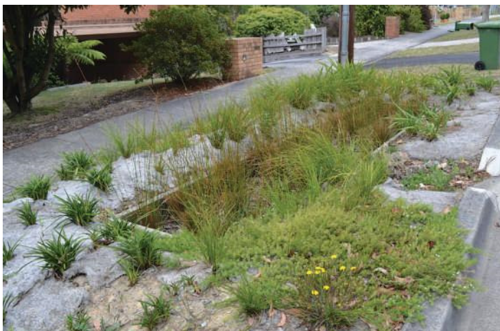
◀ Figure 3.15 Nature strip raingardens installed to filter run-off from Fernhill Road, Mount Evelyn
