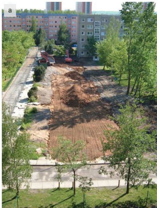
▲ Figure 8.14 (a) Apartment block demolished in Dresden 2005
