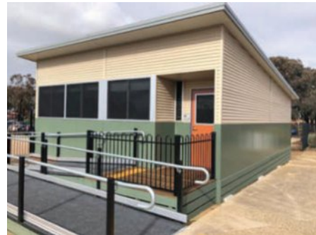
FIGURE 3.16 A purpose-built facility for the Victorian Government's Doctors in Secondary Schools program
