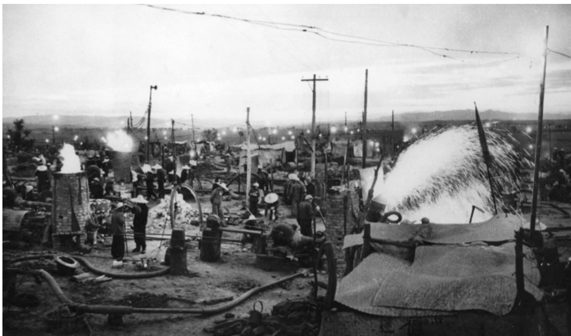
▼ Source 11.6 A steel mill during the Great Leap Forward
