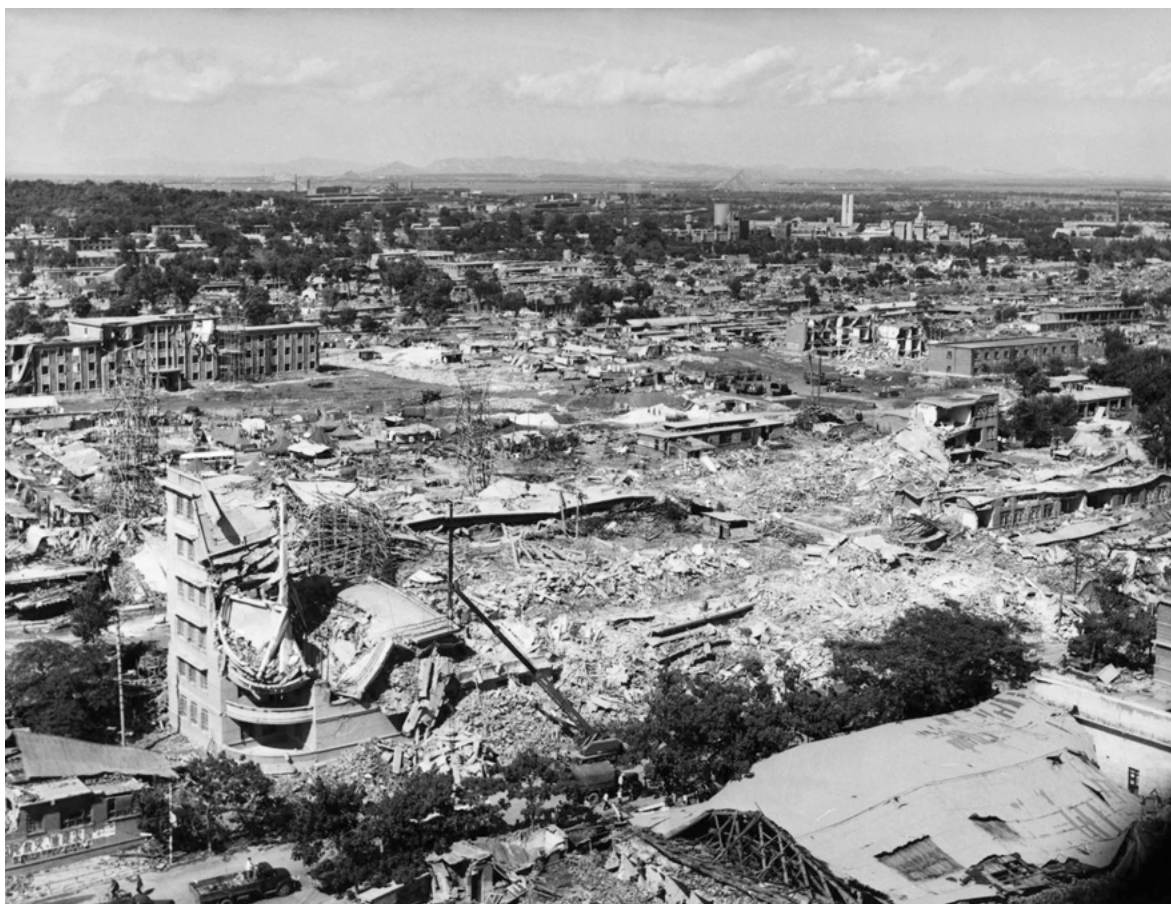
▲ Source 15.5 Aftermath of the Tangshan earthquake
