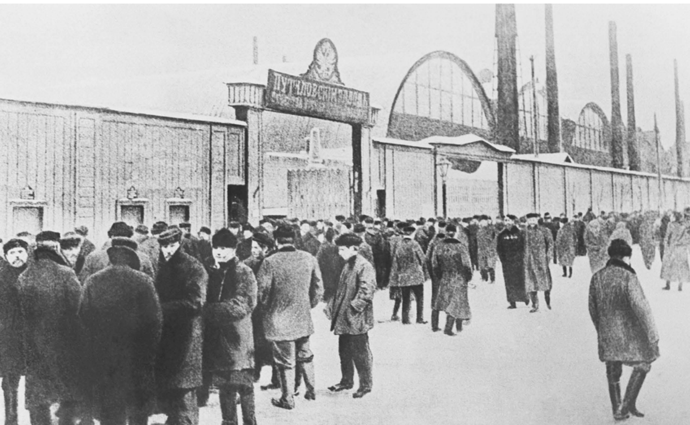
▼ Source 5.6 Strikers outside the Putilov Steel Works
