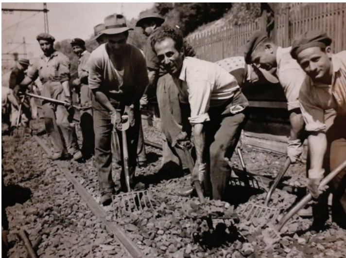
← Source 6.1 Italian migrants spreading ballast, Royal Park rail line, 1952. Courtesy State Transit Authority.
