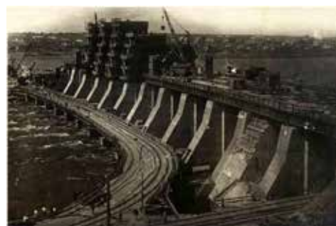
↓ Source 4.14 Construction continues on the Dnieper River Dam in Ukraine.
