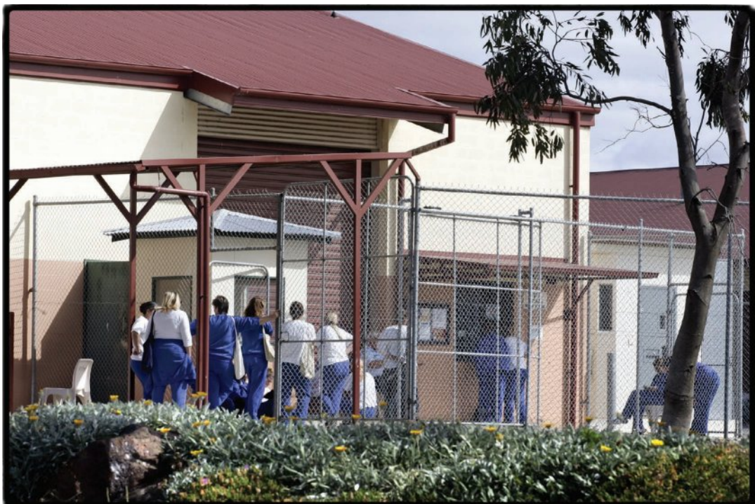
The exterior of Dame Phyllis Frost Centre, a correctional facility for women in Deer Park, Victoria.
