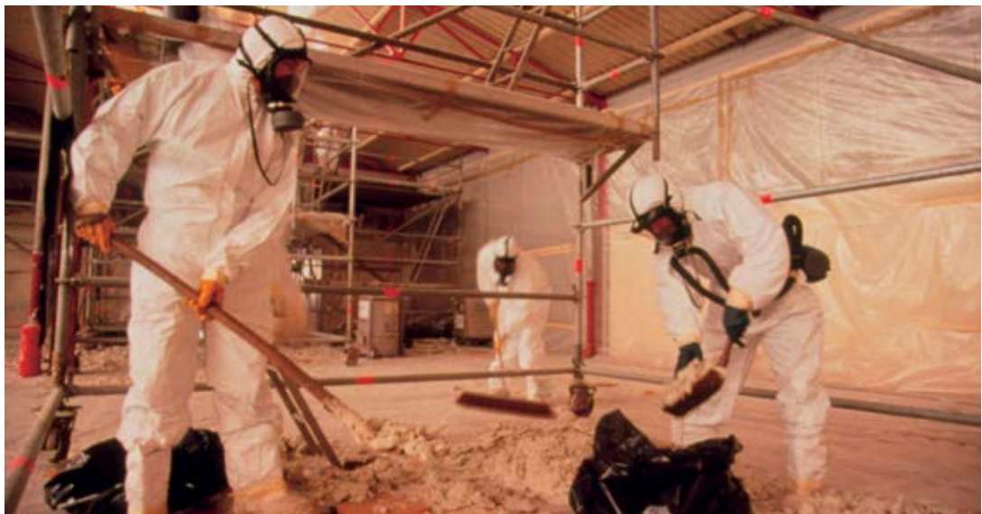
Figure 7.6 Asbestos removal requires head-to-toe protective clothing.
