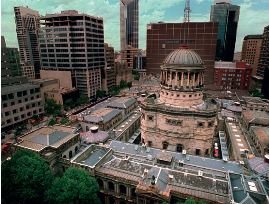
Figure 6.9 The Supreme Court of Victoria, Melbourne. The court's library is contained in the dome and all courtrooms are located around the dome.
