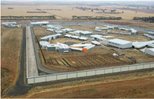
Source 1 The Melaleuca unit, HM Barwon Prison, Victoria. Barwon was the first new prison in Victoria to be designed specifically for unit management (management of small groups of prisoners by a permanent staff team).
