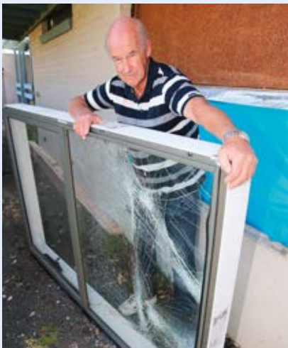
Source 4 Queenscliff renovator Geoff Morgan shows a broken window.
