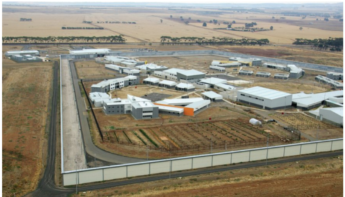
Source 1 The Melaleuca unit, HM Barwon Prison, Victoria. Barwon was the first new prison in Victoria to be designed specifically for unit management (management of small groups of prisoners by a permanent staff team).
