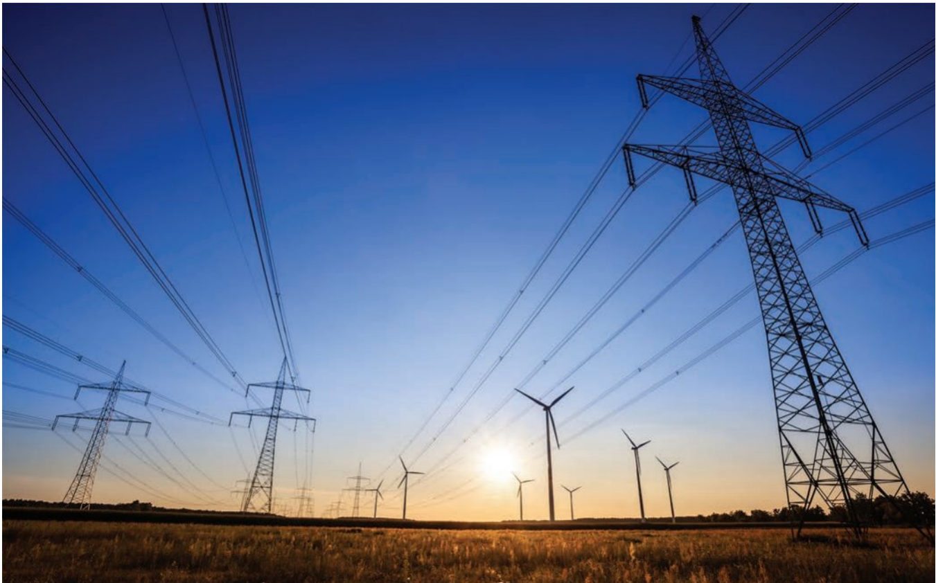
Figure 6C–1 High-voltage transmission lines carry electricity to where it is needed around Victoria and interstate. Transmission can be at 66 kV or up to 500 kV.
