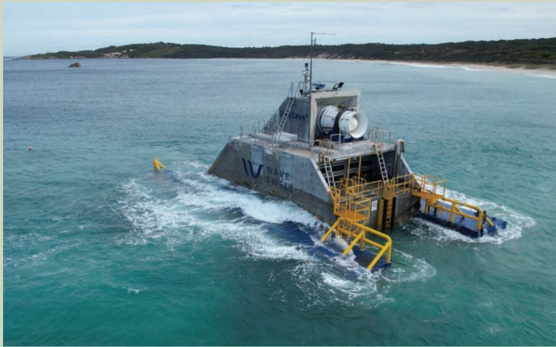
Figure 5B–2 The Uniwave OWC generator positioned in shallow water off King Island, Tasmania, where it generates electricity from wave power with 40–50% efficiency.
