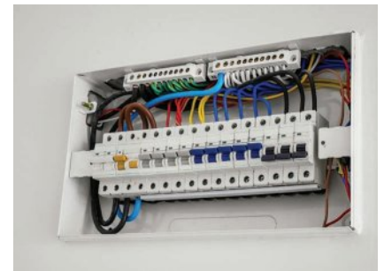
Figure 10 A consumer unit containing many RCDs
