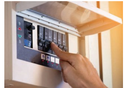
Figure 5 Resetting a 'tripped' circuit breaker
