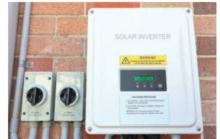
Figure 6 A solar inverter installed in a residential home
