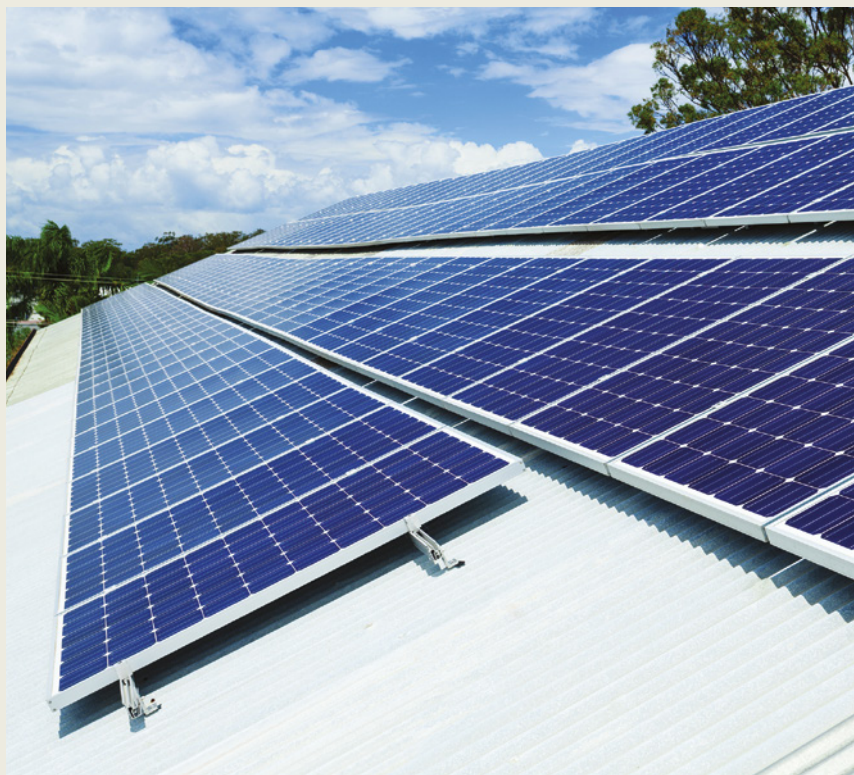
FIGURE 10.1.7 Solar panels are used to convert sunlight into electrical energy using the photoelectric effect.
