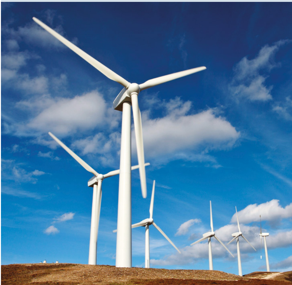
FIGURE 5.2.4 The tips of these wind-generator blades are travelling in circular paths at speeds of around 400 \text{ km h}^{-1} .
