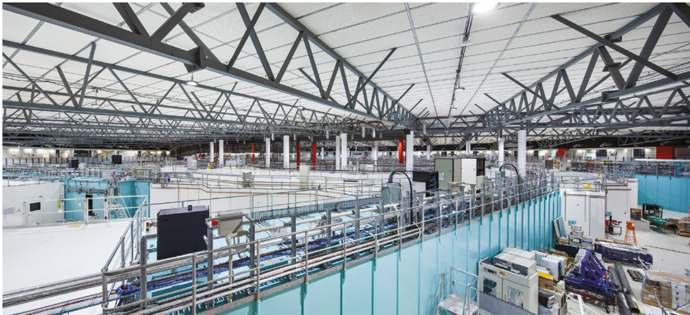
FIGURE 3.3.1 View of the inside of the Australian Synchrotron, taken from the mezzanine.
