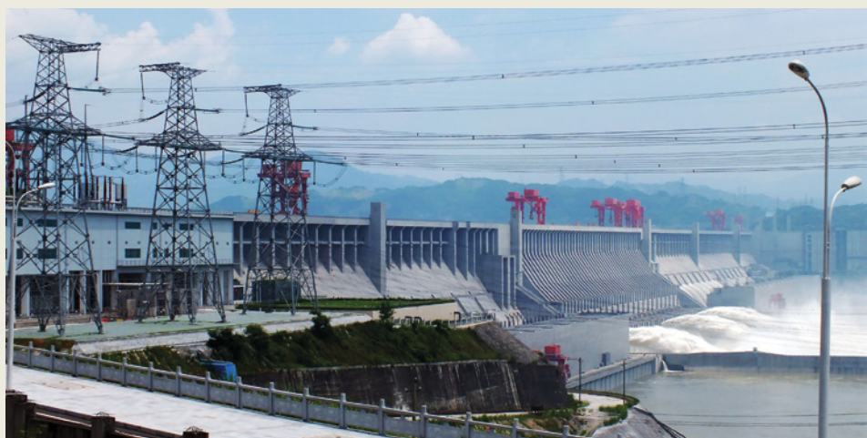
FIGURE 4.4.5 Transmitting projects at the Three Gorges Dam in China look to use DC transmission at higher voltages than is possible with AC to further reduce transmission losses.
