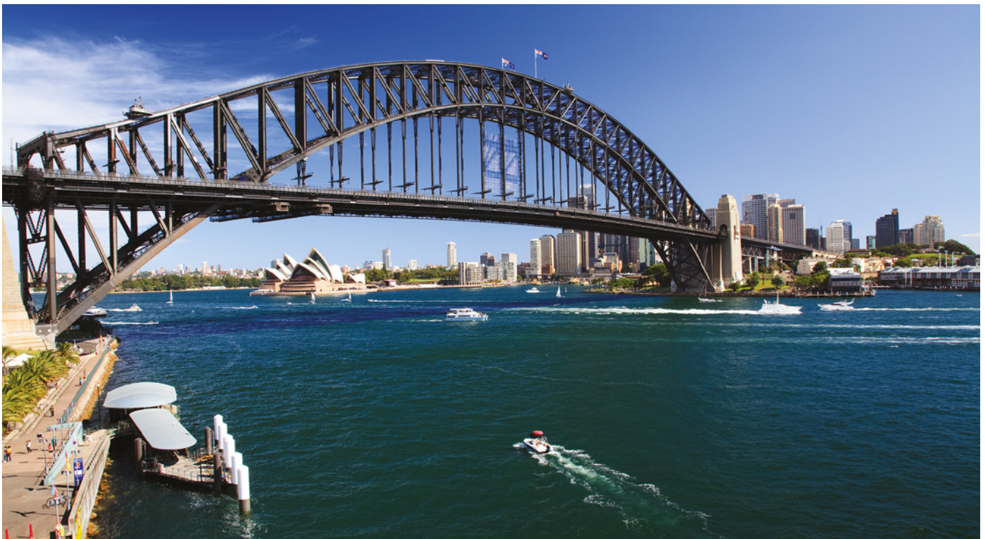
FIGURE 2.2.3 Two 1 C charges 1 m apart would produce a force of 10^{10} \text{ N} , which is almost twice the weight of the Sydney Harbour Bridge.
