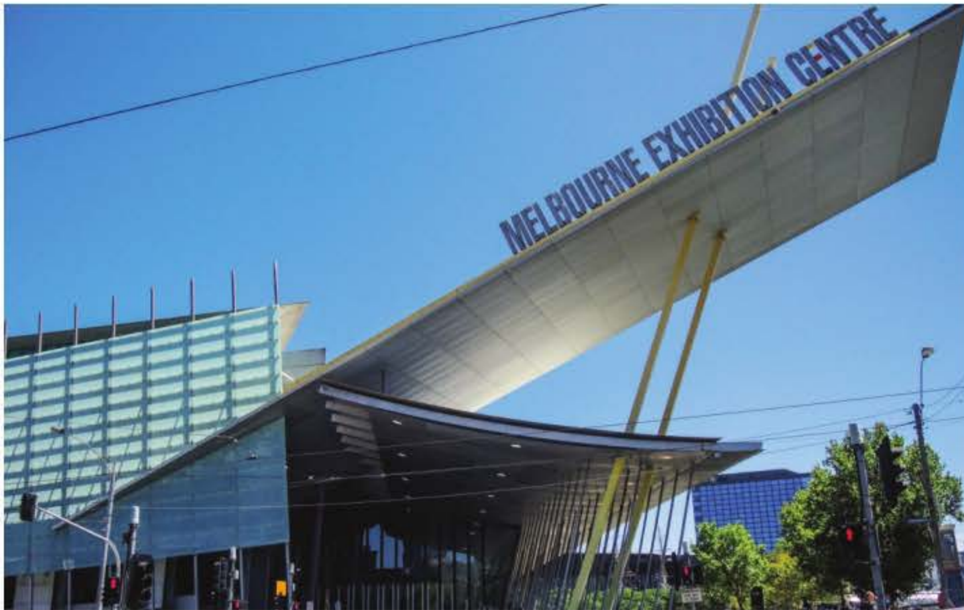
FIGURE 14.3.1 An object in translational and rotational equilibrium, like the prominent awning on the Melbourne Exhibition Centre, is in static equilibrium.
