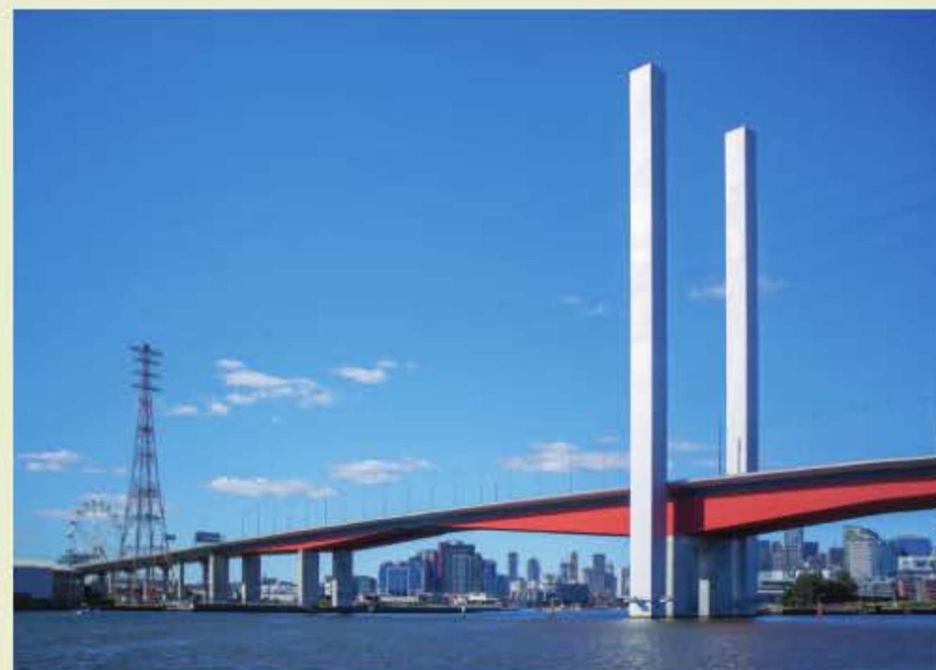
FIGURE 14.3.13 The Bolte Bridge in Melbourne is a large twin cantilever bridge. The piers are used to support different sections of road that project out horizontally.
