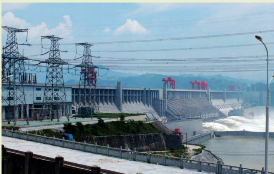
FIGURE 7.5.4 The Three Gorges Dam in China transmits DC electricity at higher voltages than is possible with AC, with an aim to reduce transmission losses.
