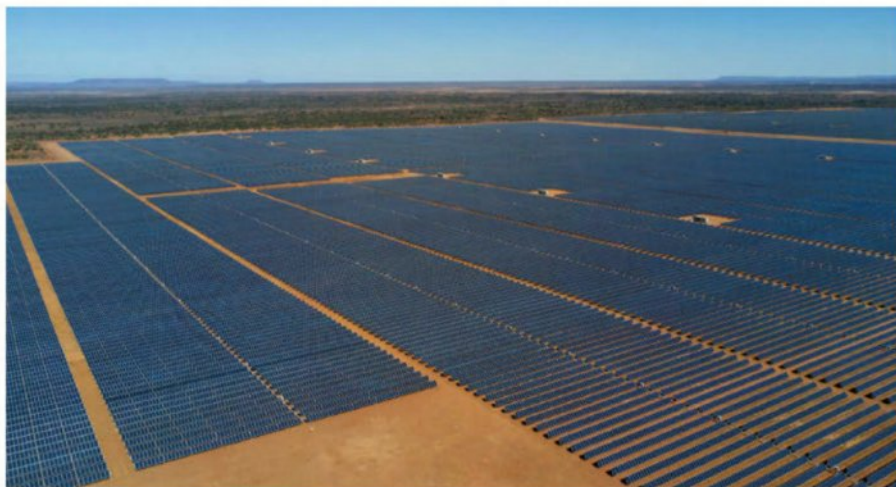
FIGURE 7.4.3 The Bungala Solar Power Project near Port Augusta, South Australia
