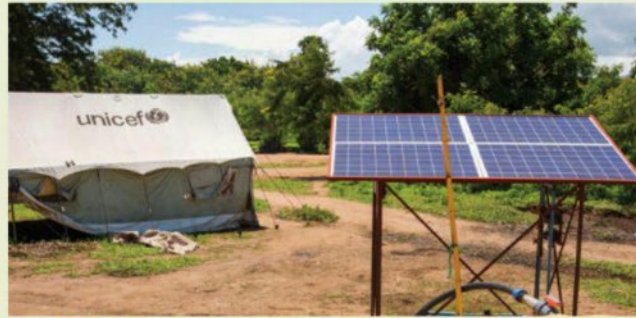
FIGURE 7.4.4 A solar-powered water pump providing an off-grid water supply for small-scale agricultural production
