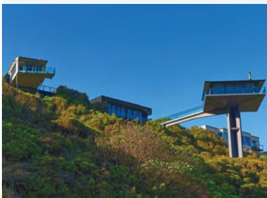
FIGURE 9.8 The Pole House located on the Great Ocean Road is supported by a concrete column that goes several metres into the ground.
