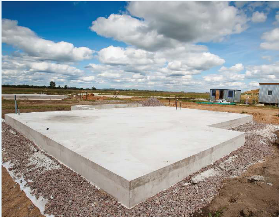
FIGURE 11.4.13 A concrete slab provides an excellent base in which to take the compressive loads of a house.
