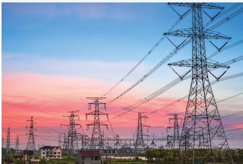
FIGURE 7.1 High-voltage power lines are used to transmit electricity over long distances.
