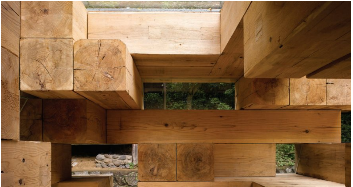
Figure 7.15 An example of joining wood for architecture, Kumamoto, Japan, Sou Fujimoto Architects, 2008
