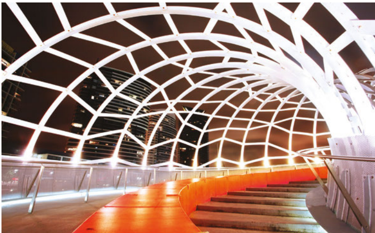
Figure 2.18 Webb Bridge in Melbourne's Docklands
