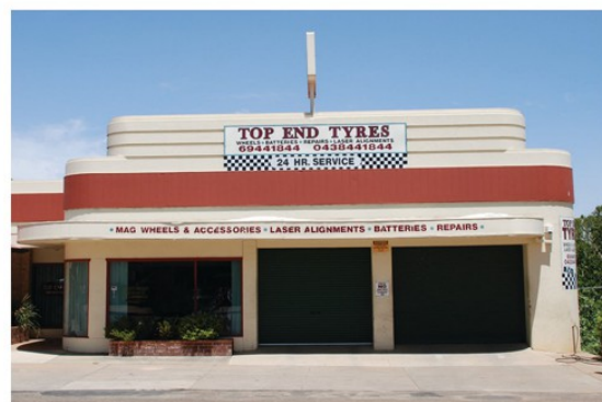
▲ Typical Australian Art Deco architecture featured rounded corners and linear details. Colours were muted and surfaces rendered or painted.
