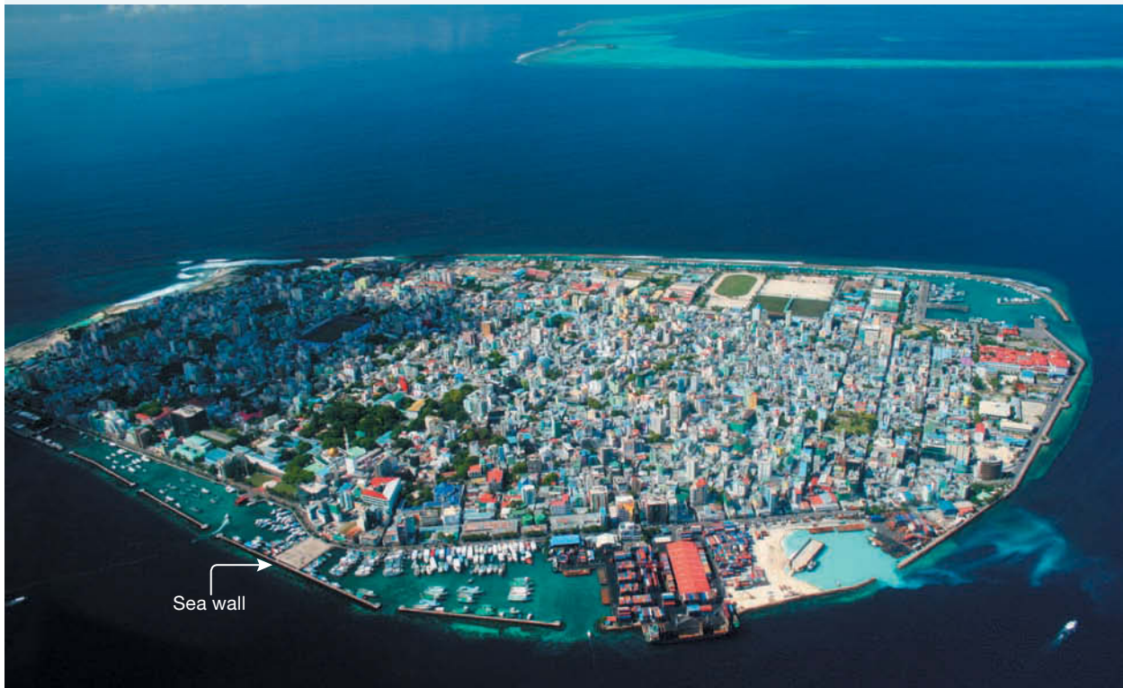
FIGURE 6 Malé, the capital of the Maldives, occupies an entire island of its own. Why is there a need for a sea wall?
