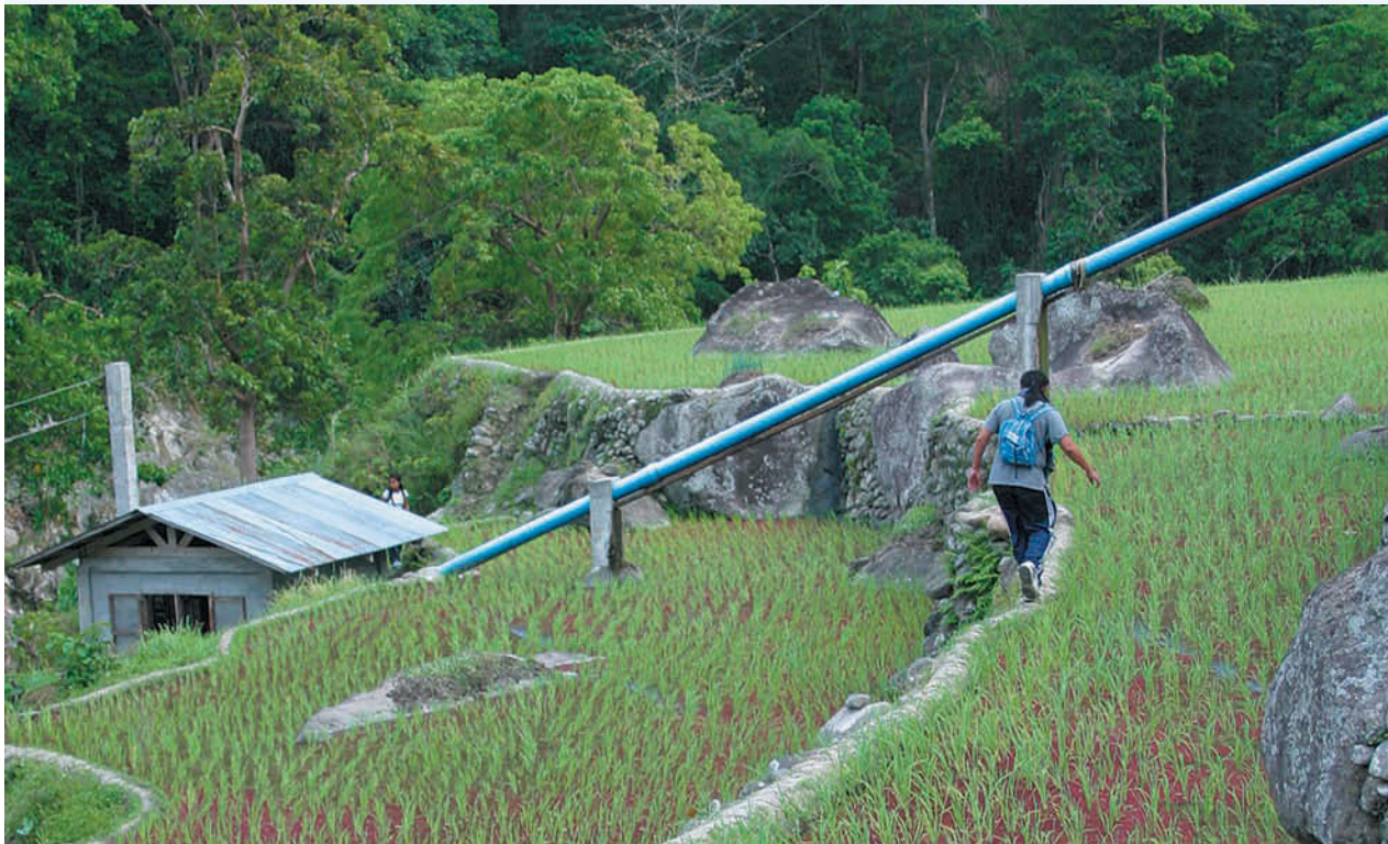
FIGURE 3 Water collected from a stream uphill rushes down the pipe and drives a small turbine in the hut to generate electricity for a local community in the Philippines.
