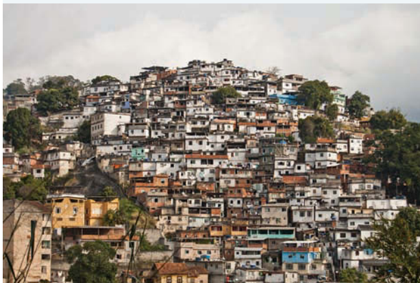
FIGURE 2 A favela located on a steep slope in Rio de Janeiro
