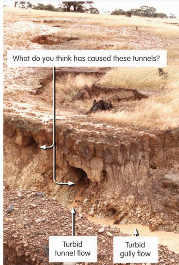
FIGURE 9 Notice that tunnel erosion forms where the surface of the land is bare. What do you think is likely to happen next?
