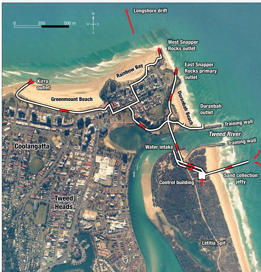
FIGURE 5 Sand bypass system
