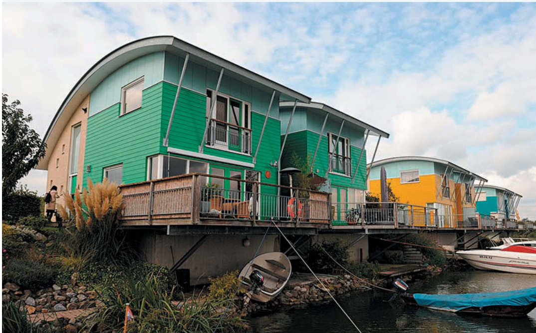
FIGURE 2 Floating settlements anchored to the embankments along the waterfront at Maasbommel, the Netherlands
