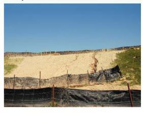
**FIGURE 3** Rill erosion. In which direction do you think the water is flowing? Why?
