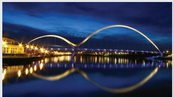
This image shows why the Infinity Bridge, England, is named after the symbol \infty . Architects develop and solve equations in three dimensions to determine the intersection points of lines (support cables) and parabolic curves (the arches).
