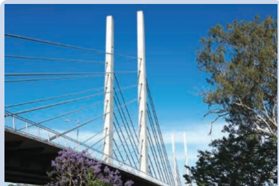
The Eleanor Schonell Bridge in Brisbane is a cable-stayed bridge in which each cable forms a right-angled triangle with the pylons and the bridge deck. Trigonometry and geometry are essential tools for engineers.
