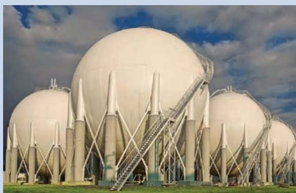
Spherical tanks store compressed or liquid gases for the petroleum and chemical industries. The spherical shape uses the smallest land area for the storage volume and distributes pressure evenly over the sphere's surface area.
