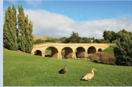
Richmond Bridge, Tasmania, is the oldest bridge in Australia that is still in use.
