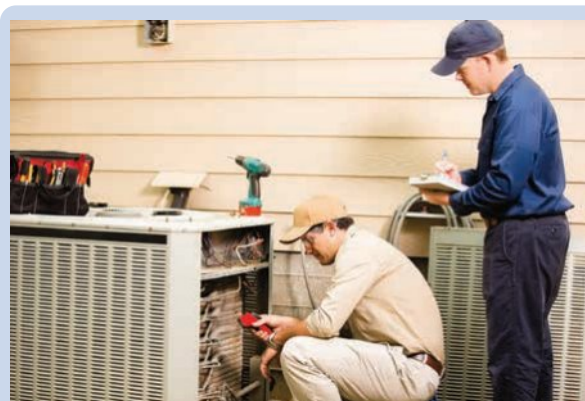
The study of air-conditioning uses algebraic fractions to model airflow, air temperatures and humidity. The mechanical engineers who design ventilation systems, and the electricians who install and repair them, all require algebraic skills.
