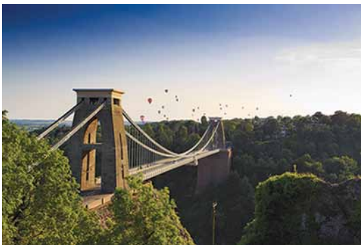
The cables from a suspension bridge
