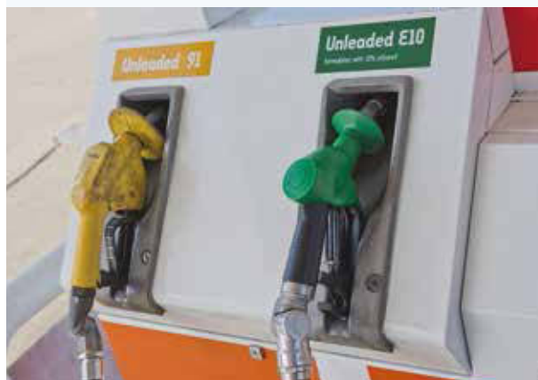
FIGURE 5.28 E10 is a blend of 10 per cent ethanol and 90 per cent unleaded petrol
