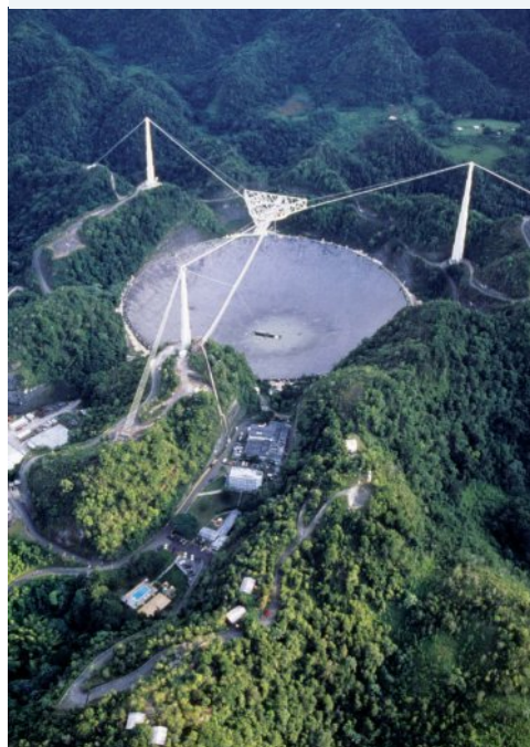
FIGURE 6.19 The Arecibo dish in Puerto Rico was the largest single radio telescope in the world. It is 305 metres across.
