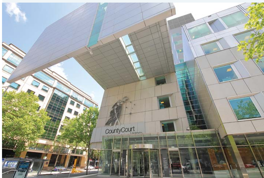
FIGURE 1 Victoria's County Court
