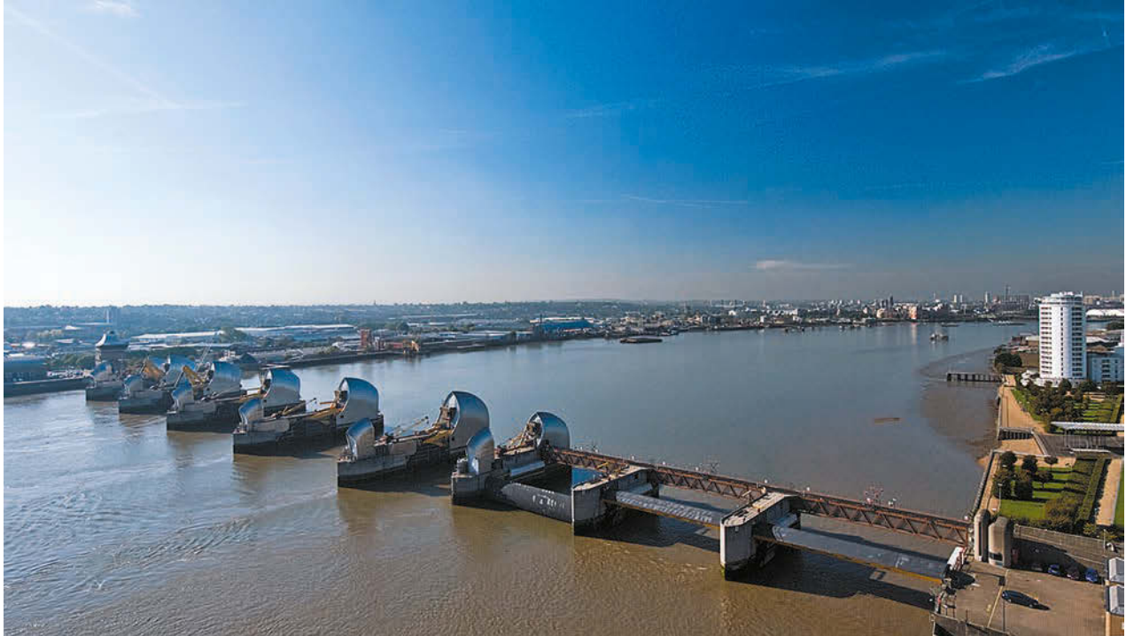
FIGURE 3 The Thames flood barrier seen here with its gates up
