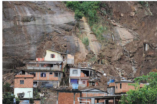
FIGURE 7 Hills collapsed after the heavy rains, destroying homes.
