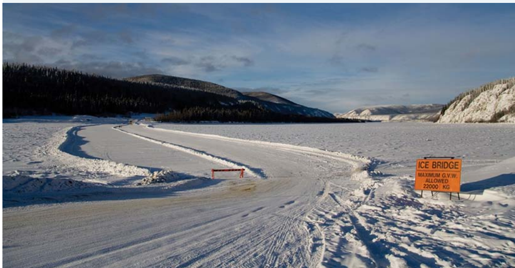
FIGURE 3 It is so cold in winter that the Yukon River freezes over, and the ice is thick enough to support fully loaded trucks.
