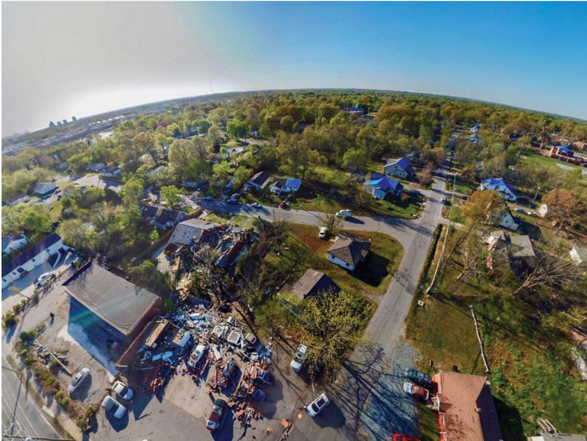
FIGURE 4 In April 2018 in Greensboro, North Carolina, trees were ripped from the ground, buildings flattened and electricity cut when a tornado carved a 54-kilometre path of destruction through the township. Wind speeds in excess of 217 kph were recorded.
