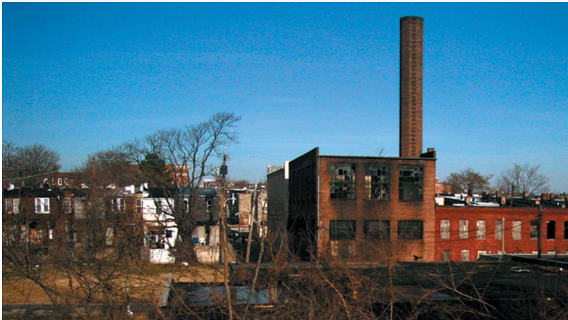
FIGURE 3 A disused factory near Baltimore
