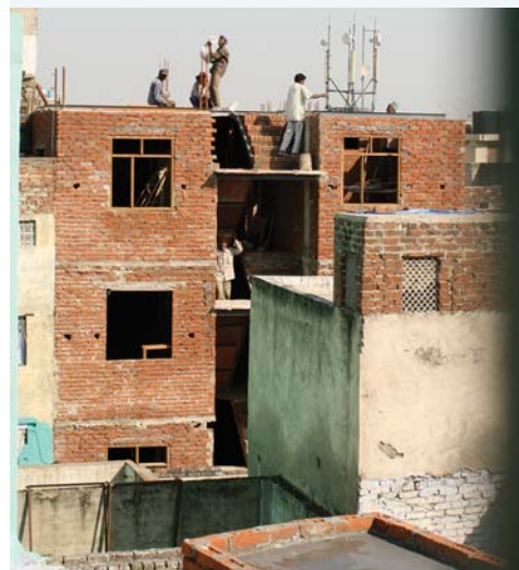
FIGURE 1 Building a new multi-storey building inside Old Delhi
