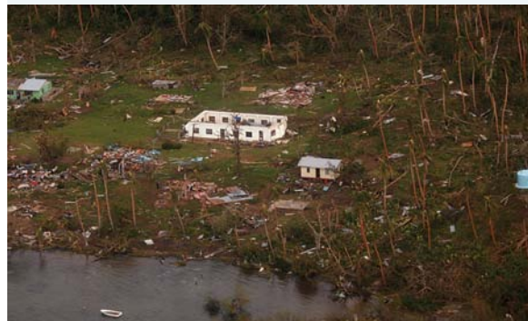
FIGURE 8 Additional damage was caused by a 4-metre storm surge.
