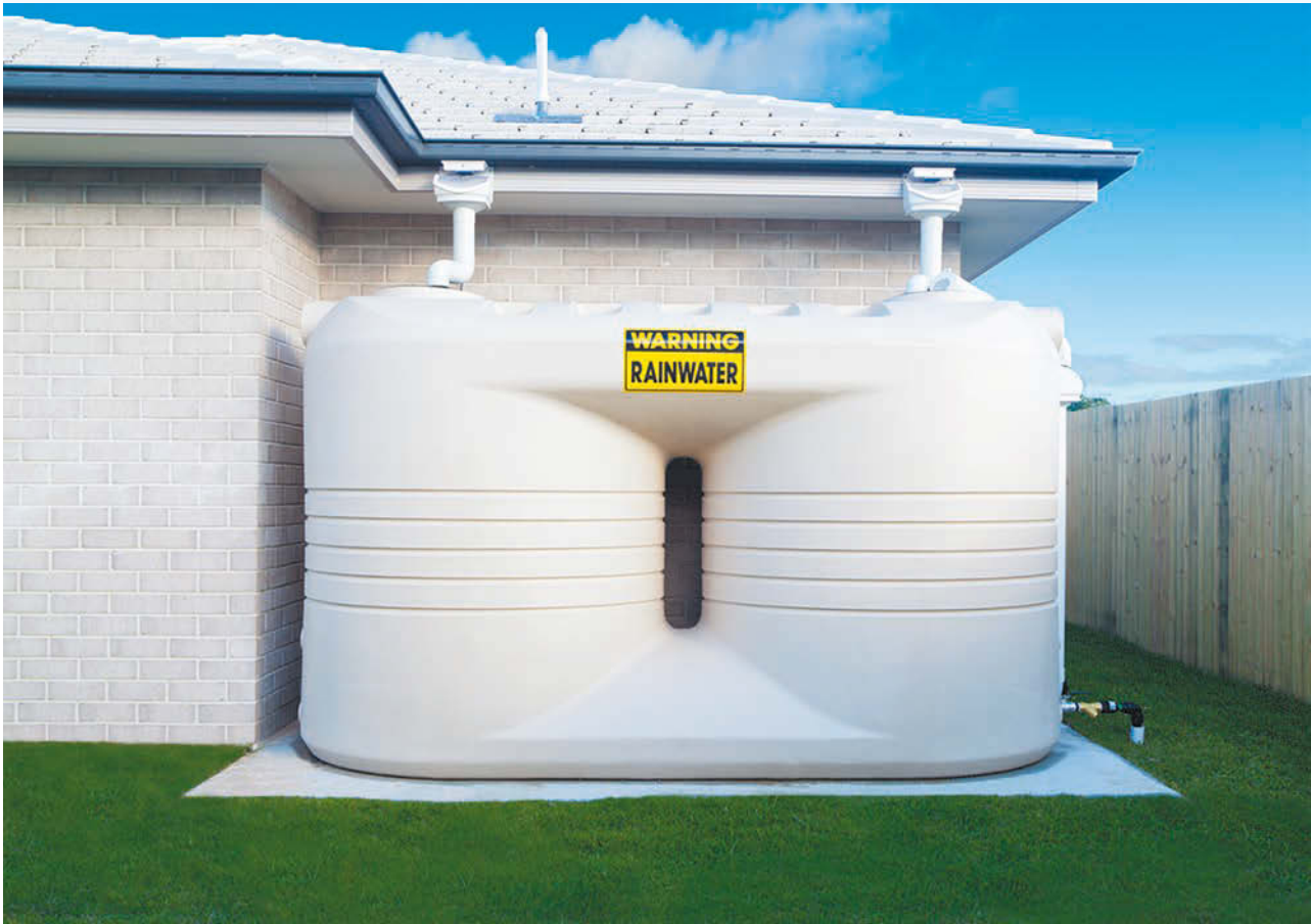
FIGURE 3 Collecting rainwater from your roof can provide water for flushing toilets, watering the garden or washing the car.
