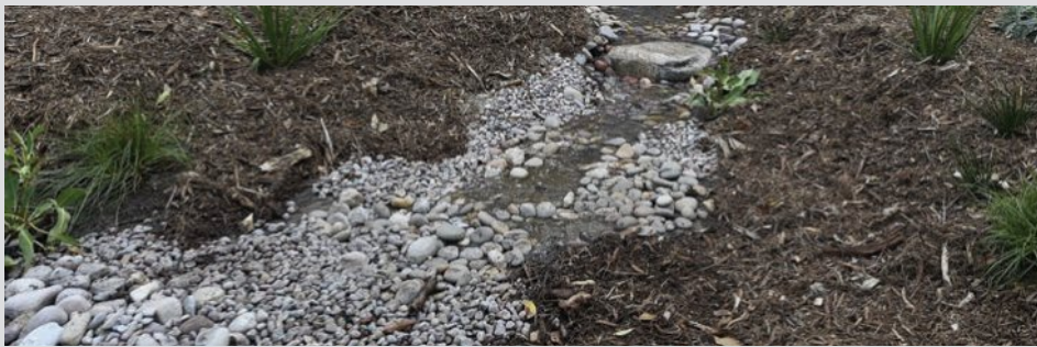
▲ Figure 7.44 Stormwater runoff is directed into this raingardens like this one so that water can filter into the ground rather than flooding local creeks
