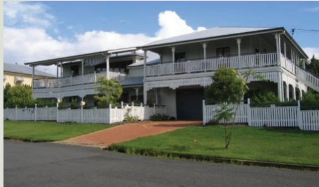
▲ Figure 10.24 Traditional Queenslanders are built raised from the ground to counteract flooding and encourage a cooling airflow
