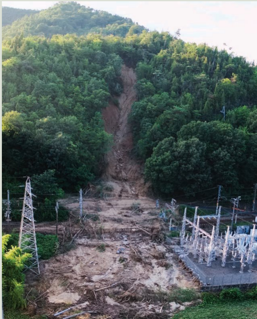
▲ Figure 9.25 This landslide in Hiroshima prefecture that was triggered by the 2018 flooding in western Japan. The landslide covered the railway lines and brought down powerlines.
