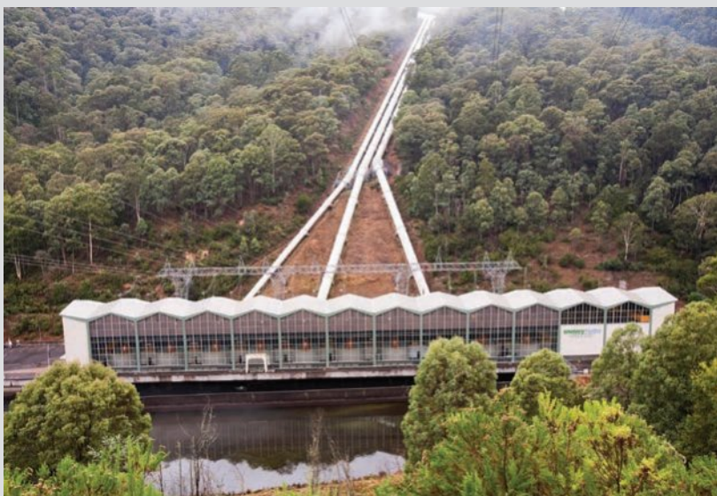
◀ Figure 7.35 Regulating the flow of rivers can be used to generate electricity. The Snowy Mountains Hydro Scheme has 10 turbine generators and each one can generate enough electricity to power 95 000 homes.
