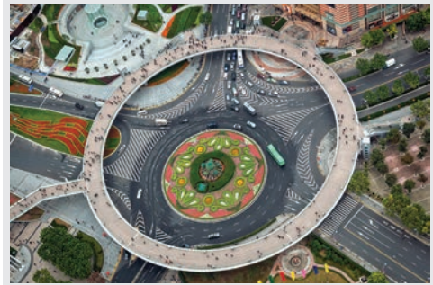
Engineers apply circle geometry when designing road roundabouts and flyovers. This image from Shanghai shows a circular pedestrian roundabout constructed above a vehicle roundabout.
