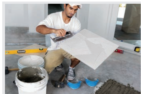
On a 20 kg bag of dry tiling adhesive the manufacturer's instructions might be to mix the 20 kg with 7.5 litres of water. A tiler can simplify this rate to a more suitable rate of 750 mL water/2 kg of tile adhesive.
