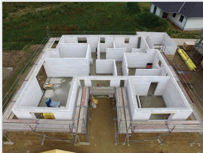
The perimeter of a house is found by adding the lengths of all the outside walls. Scaffolding is required around the perimeter for construction work above ground level.
