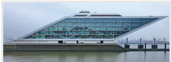
The architect has used a parallelogram to design this office building in Hamburg, Germany. The steel structural supports linking the sides form rhombus shapes and triangles.
