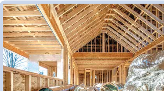
A builder makes sure that the roof rafters are all parallel, the ceiling joists are horizontal and parallel, and the wall studs are perpendicular and parallel.
