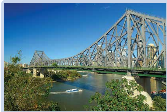
Engineers calculate the angles between the straight structural supports used on bridges such as the angles seen here on the Story Bridge, Brisbane.
