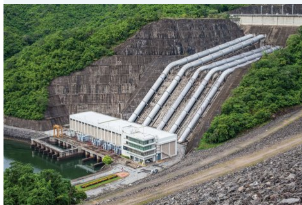
FIGURE 7.19 In a hydroelectric power station the turbines are driven by water falling through pipes from a high dam.
