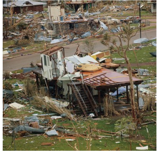
FIGURE 7.24 Cyclone Tracy devastated Darwin on Christmas Eve in 1974. It killed 65 people and injured 650. Nearly 70 per cent of homes were destroyed.
