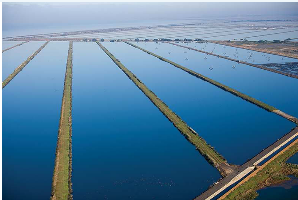
FIGURE 5.30 The lagoon system at Melbourne Water's Western Treatment Plant in Werribee
