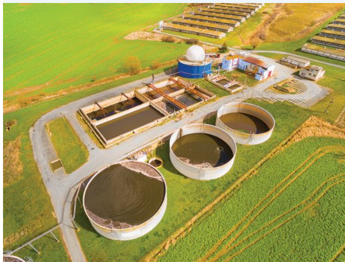
FIGURE 7.15 A biogas plant at a pig farm in the Czech Republic producing renewable energy from biomass.
