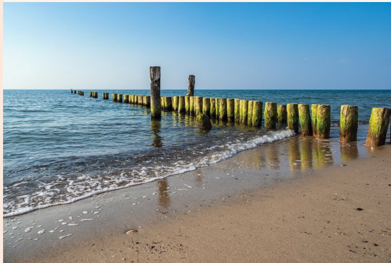
FIGURE 7.35 An example of a groyne built as a barrier
