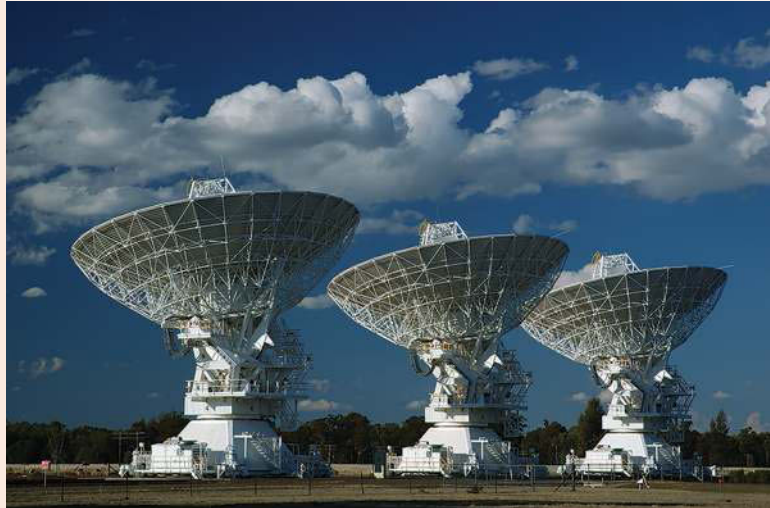
FIGURE 6.26 CSIRO's Australia Telescope Compact Array near Narrabri, NSW, built in 1988, consists of radio telescopes that can be moved along railway tracks to make a more complete picture of the sky. (Photograph courtesy of CSIRO).
