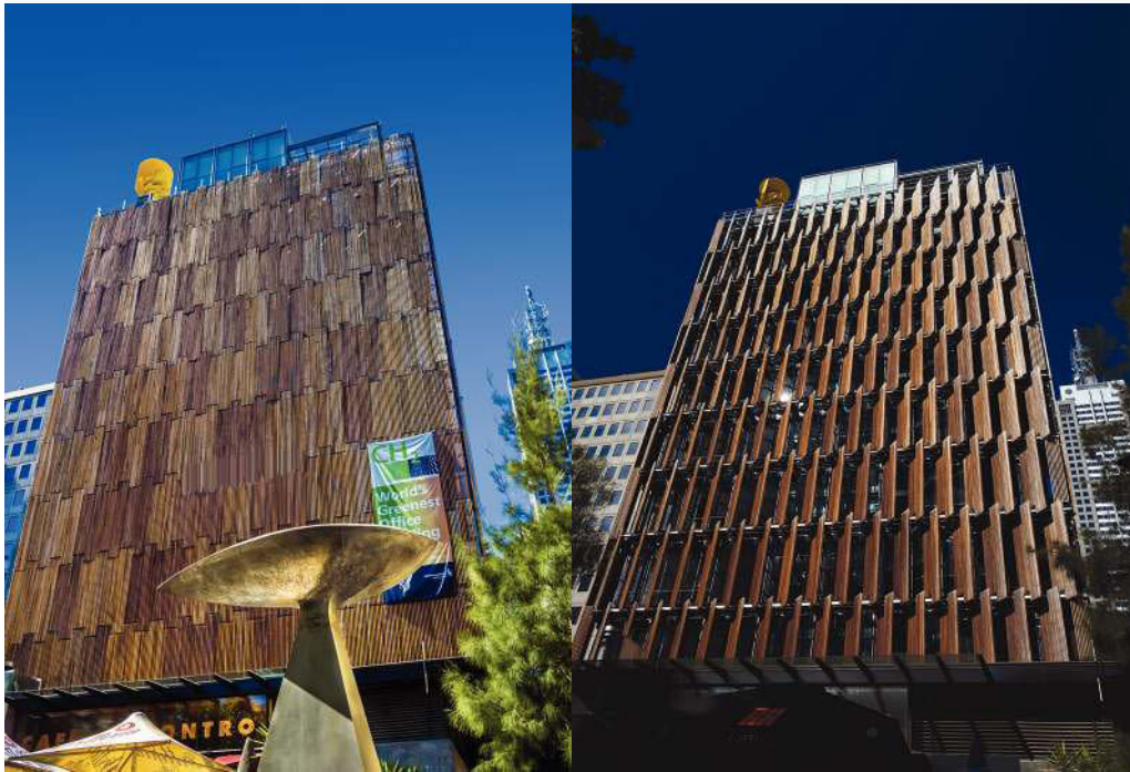
FIGURE 1 Council House 2 in Melbourne was the first Australian building to be awarded a six-star green rating. Its features include a green roof and louvred shading system.
