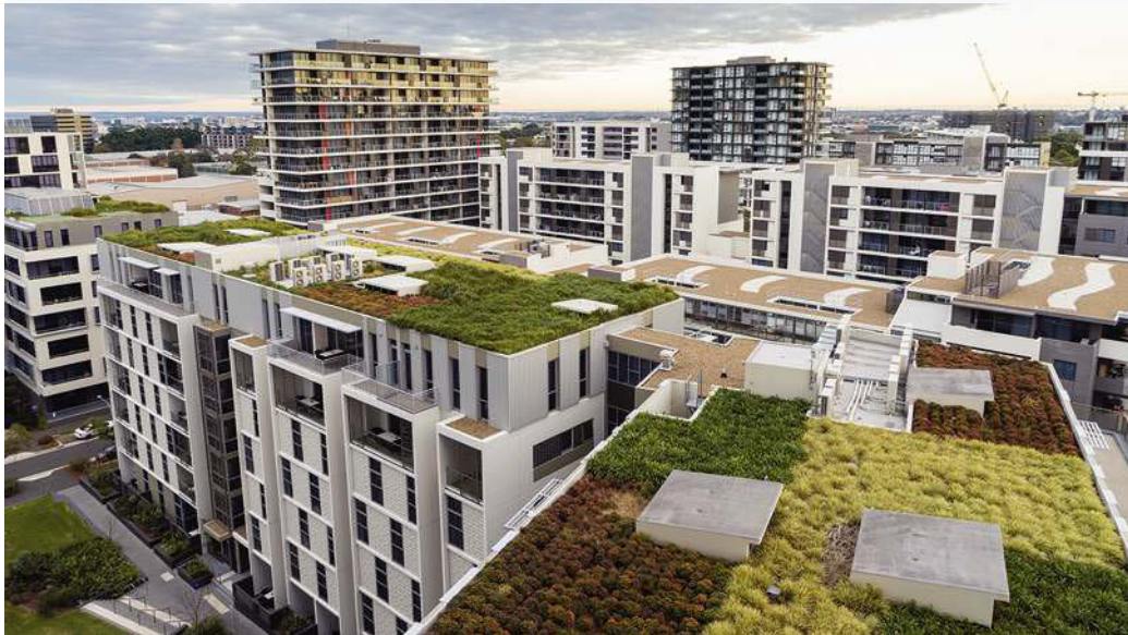
FIGURE 4 Green roof design on apartment buildings in Sydney's Pyrmont.
