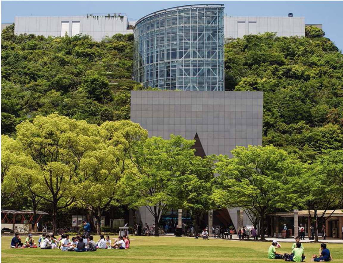
FIGURE 3 The ACROS Fukuoka building located in Fukuoka, Japan
