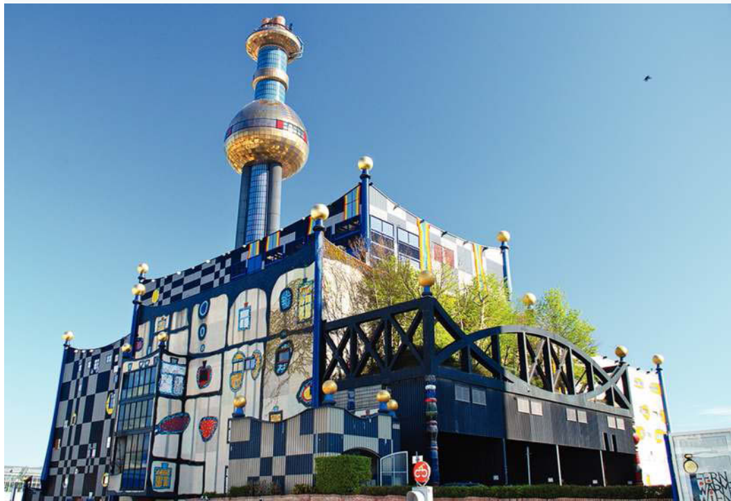
FIGURE 5 Spittelau waste treatment plant in Vienna, Austria. This power station burns waste, thus reducing landfill, to produce heat that is supplied to thousands of buildings.
