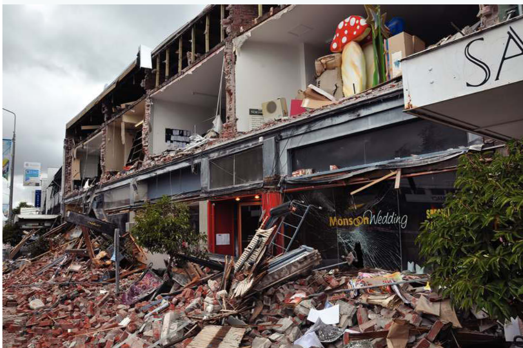
FIGURE 5 Earthquake damage in Christchurch
