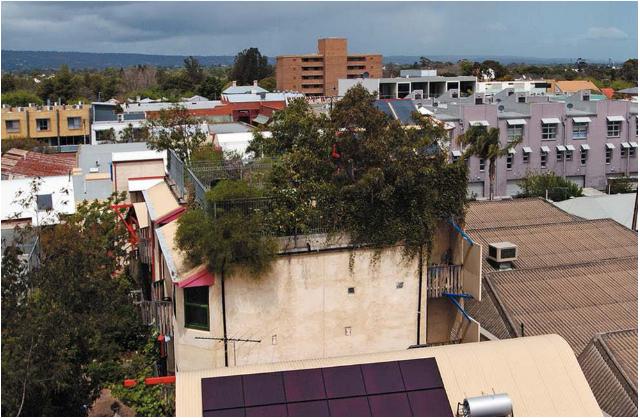
FIGURE 6 Rooftop gardens provide good insulation, protecting the buildings below from the hot sun in summer. In winter, they keep warmth from escaping from the building below.
