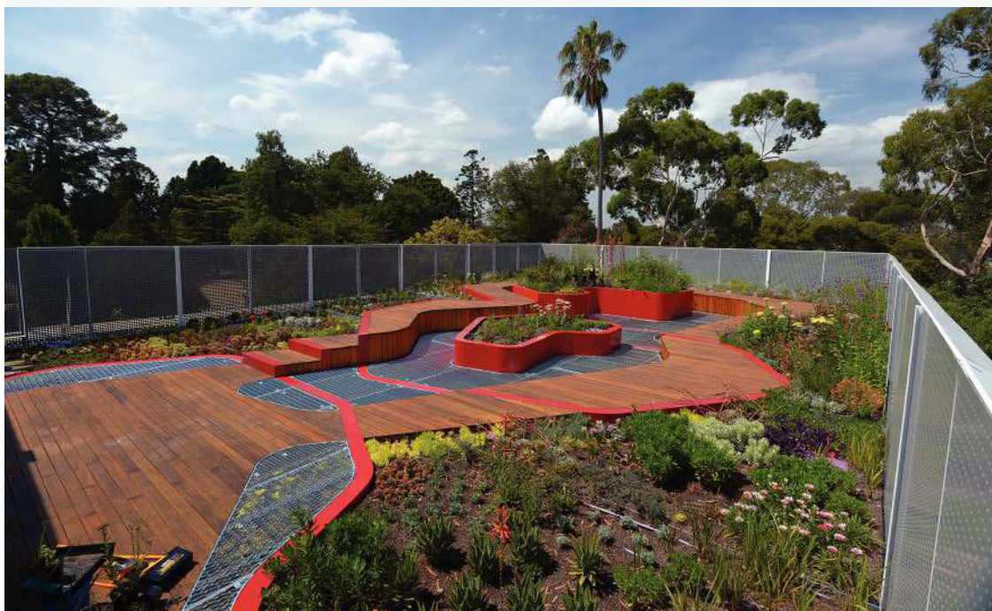
FIGURE 2 The Burnley Living Roof at the University of Melbourne's Burnley Campus
