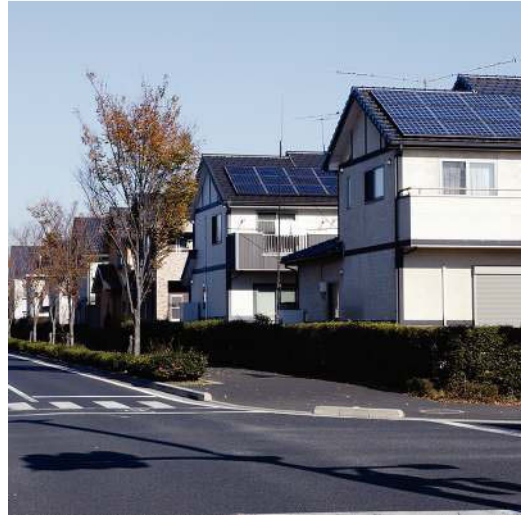
FIGURE 4 A street in Ota, Japan — solar panels are visible on most of the houses.
