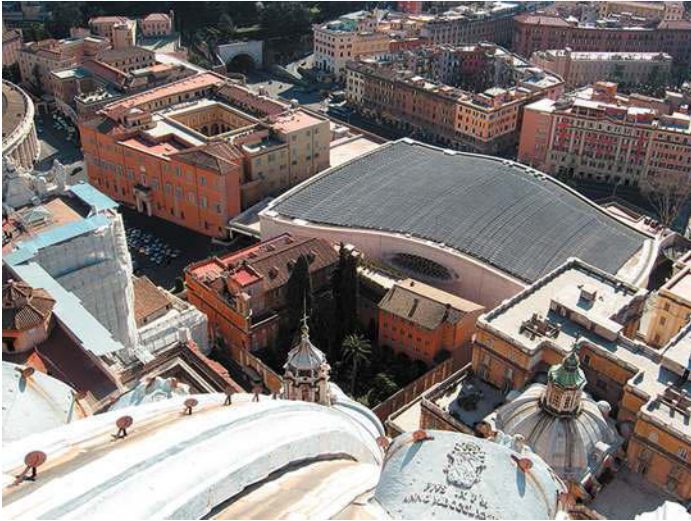
FIGURE 3 Solar panels cover the roof of the Paul VI Hall, as seen from the dome of St Peter's Basilica.
