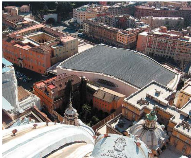
FIGURE 9 The Vatican is the world's smallest independent state. In 2008 more than 2000 photovoltaic panels were fixed to the roof of one of the city state's main buildings — the roof of the Paul VI Hall — enabling the Vatican to cut its carbon dioxide emissions by about 225 tonnes a year. The 2400 panels heat, light and cool the hall and several surrounding buildings, producing 300 kilowatt hours (MWh) of clean energy a year.
