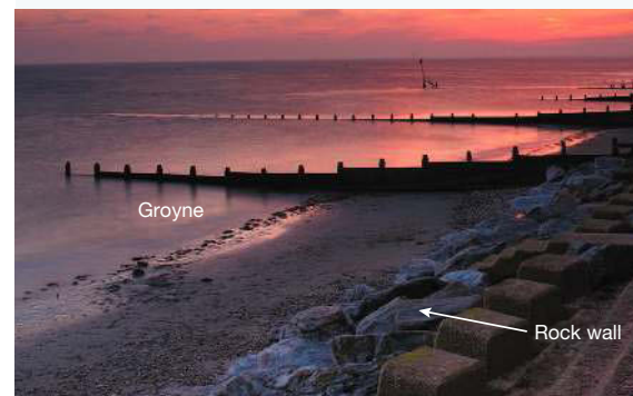
FIGURE 5 A groyne and rock barrier protect a sandy beach in Wales, United Kingdom.
